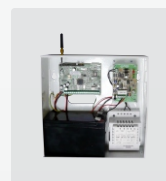
POWER SUPPLY BACKUP BATT BOX
